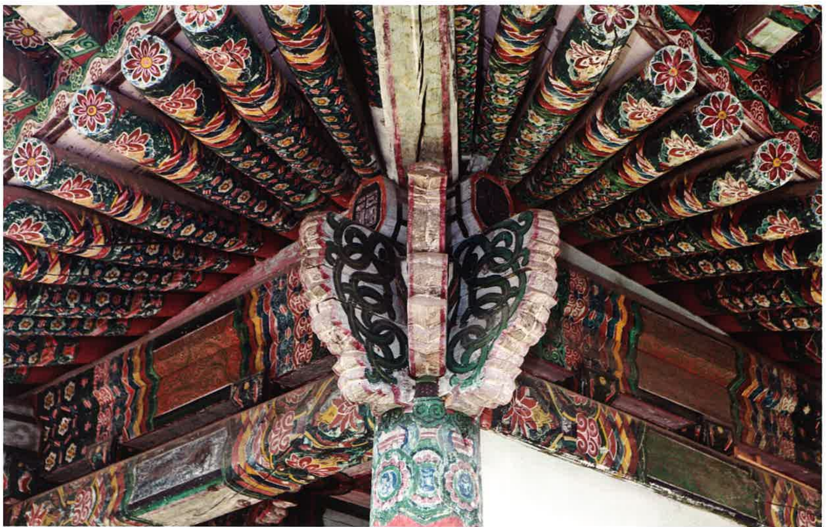
만수각 귀포 / 柱上包 耳包 / corner brackets, Mansugak
