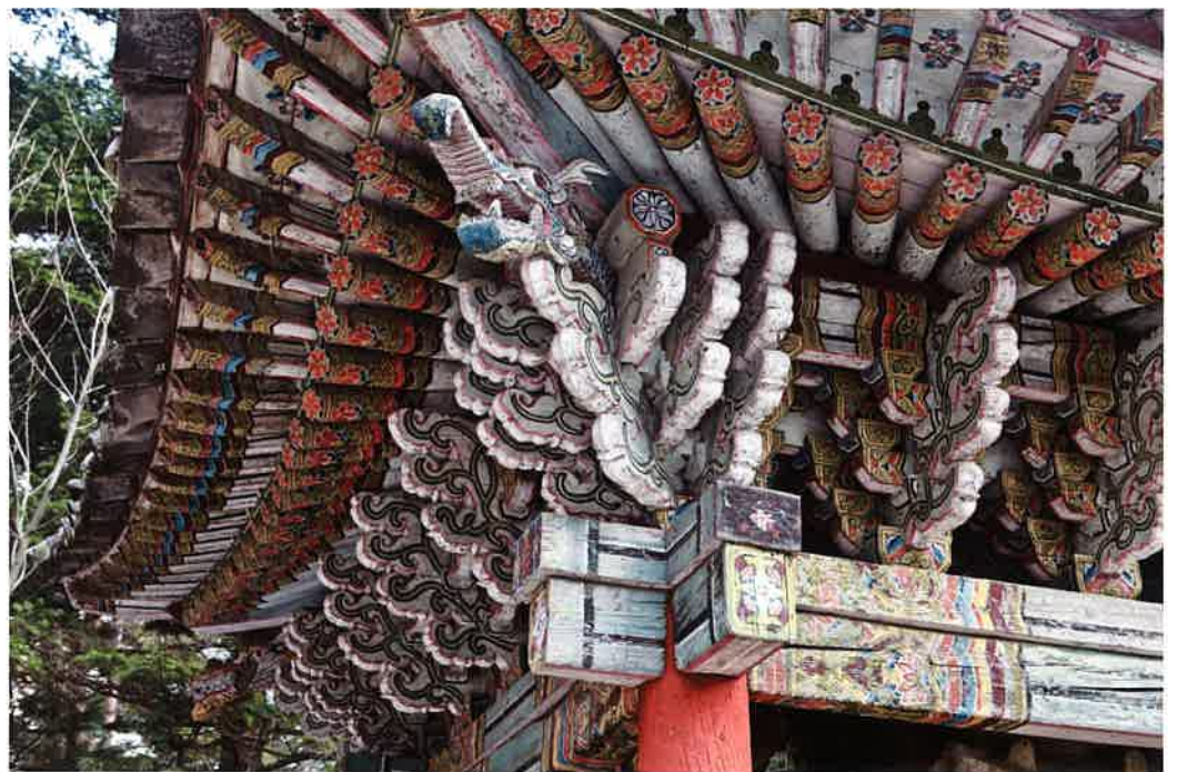
수충사 비각 귀포 / 酬忠祠 碑閣 耳包 / corner brackets of pavilion for the stone monument, Such'ungsa
