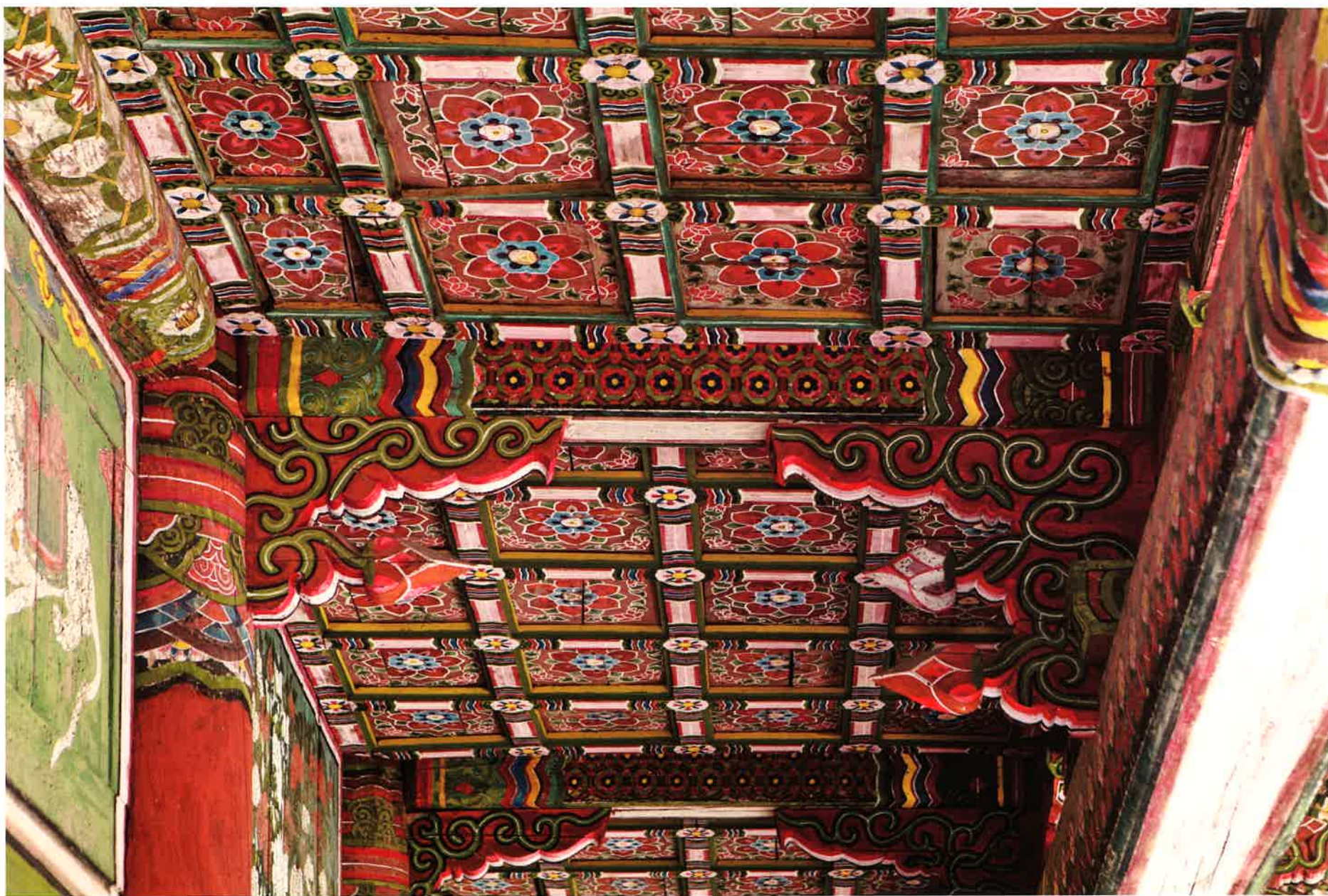
관음전 뒷간 공포와 반자 / 觀音殿 退間 栱包·天障 / brackets and ceiling of space with extra poles outside the inner fence, Kwanŭmjŏn hall
