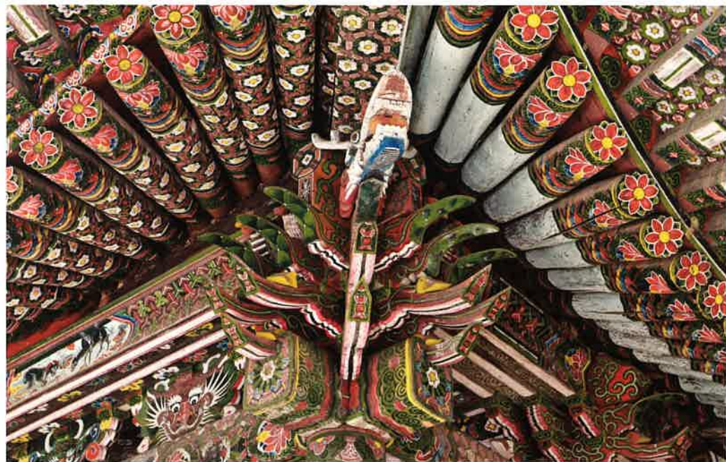
관음전 앞면 귀포 / 觀音殿 前面 耳包 / front corner brackets, Kwanŭmjŏn hall
