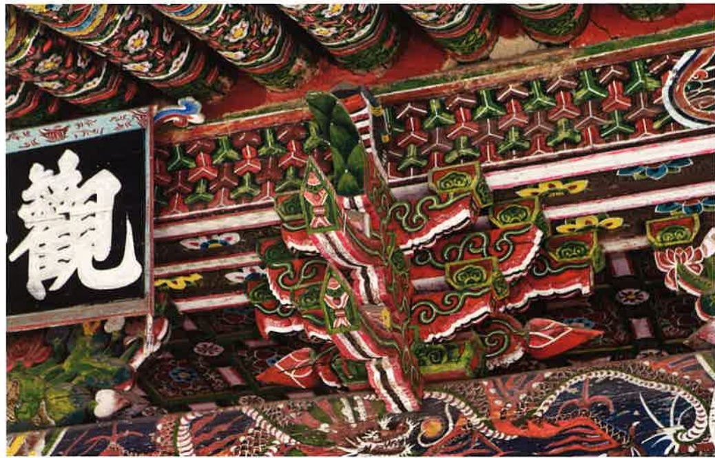
관음전 앞면 주간포 / 觀音殿 前面 柱間包 / brackets between front columns, Kwanŭmjŏn hall
