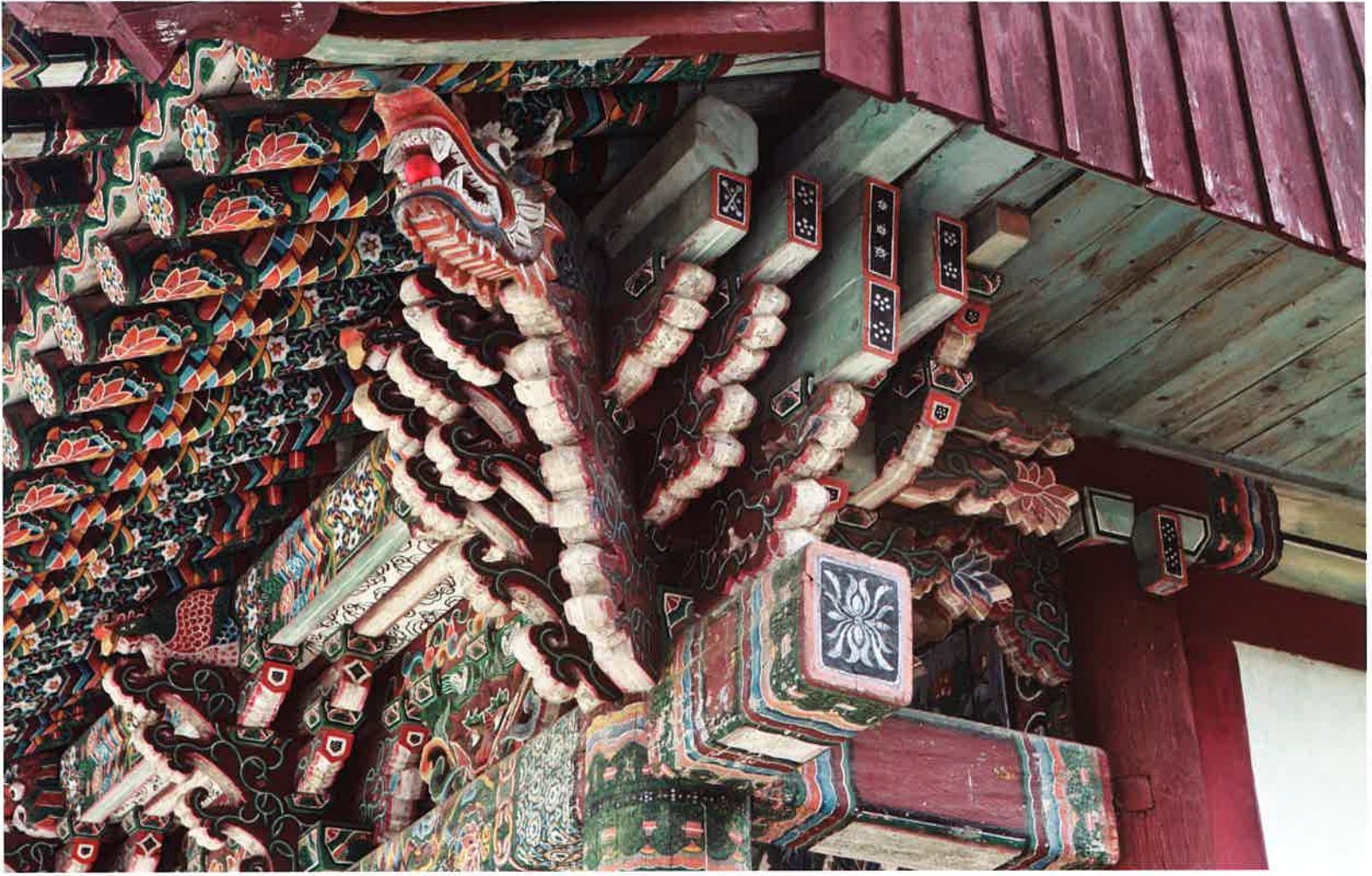
영산전 앞면 동쪽 귀포 / 靈山殿 前面 東側 耳包 / front eastern corner brackets, Yongsanjön hall
