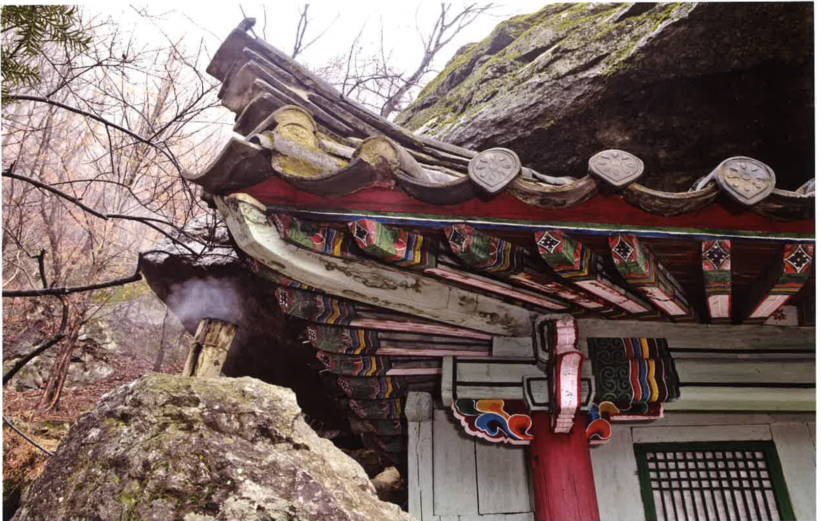
금강암 서쪽 추녀 / 金剛庵 西側 春舌 / western corners of eaves, Kūmgangam
