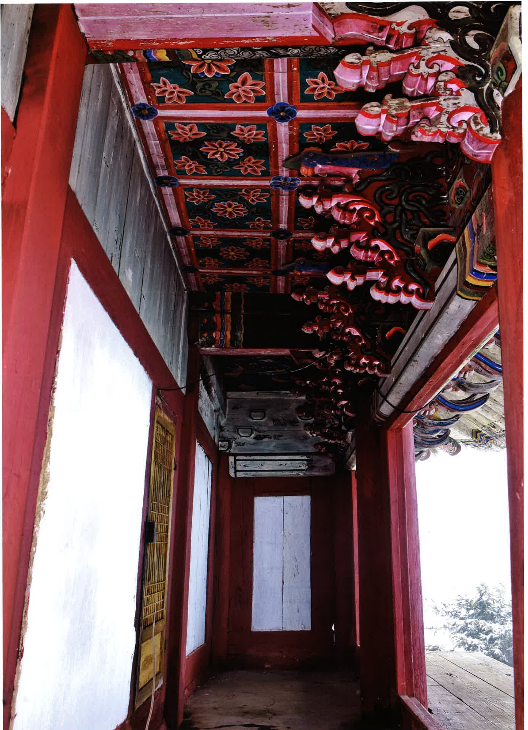
능인암 뒷간 / 能仁庵 退間 / space with extra poles outside the inner fence, Nūnginam
