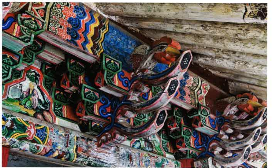
능인암 앞면 주간포 / 能仁庵 前面 柱間包 brackets between front columns, Nügingnam
