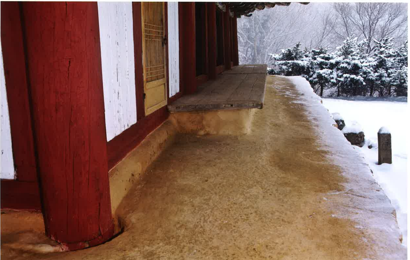
능인암 앞면 윗마루 / 能仁庵 前面 退抹樓 / front narrow wooden porch running along the outside of a room, Nūnginam
