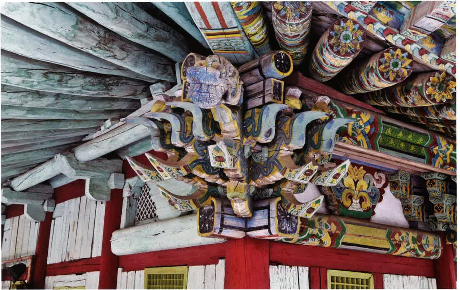
불영암 뒷면 서쪽 귀포 / 佛影庵 後面 西側 耳包 / backward western corner brackets, Puryongam
