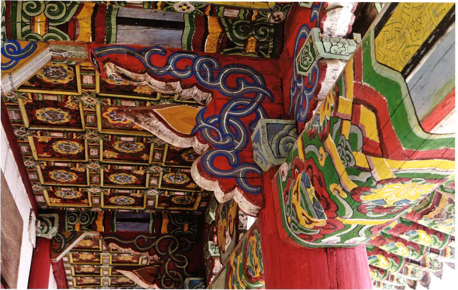
불영암 뒷간 공포 / 佛影庵 退間 栱包 / brackets of space with extra poles outside the inner fence, Puryŏngam
