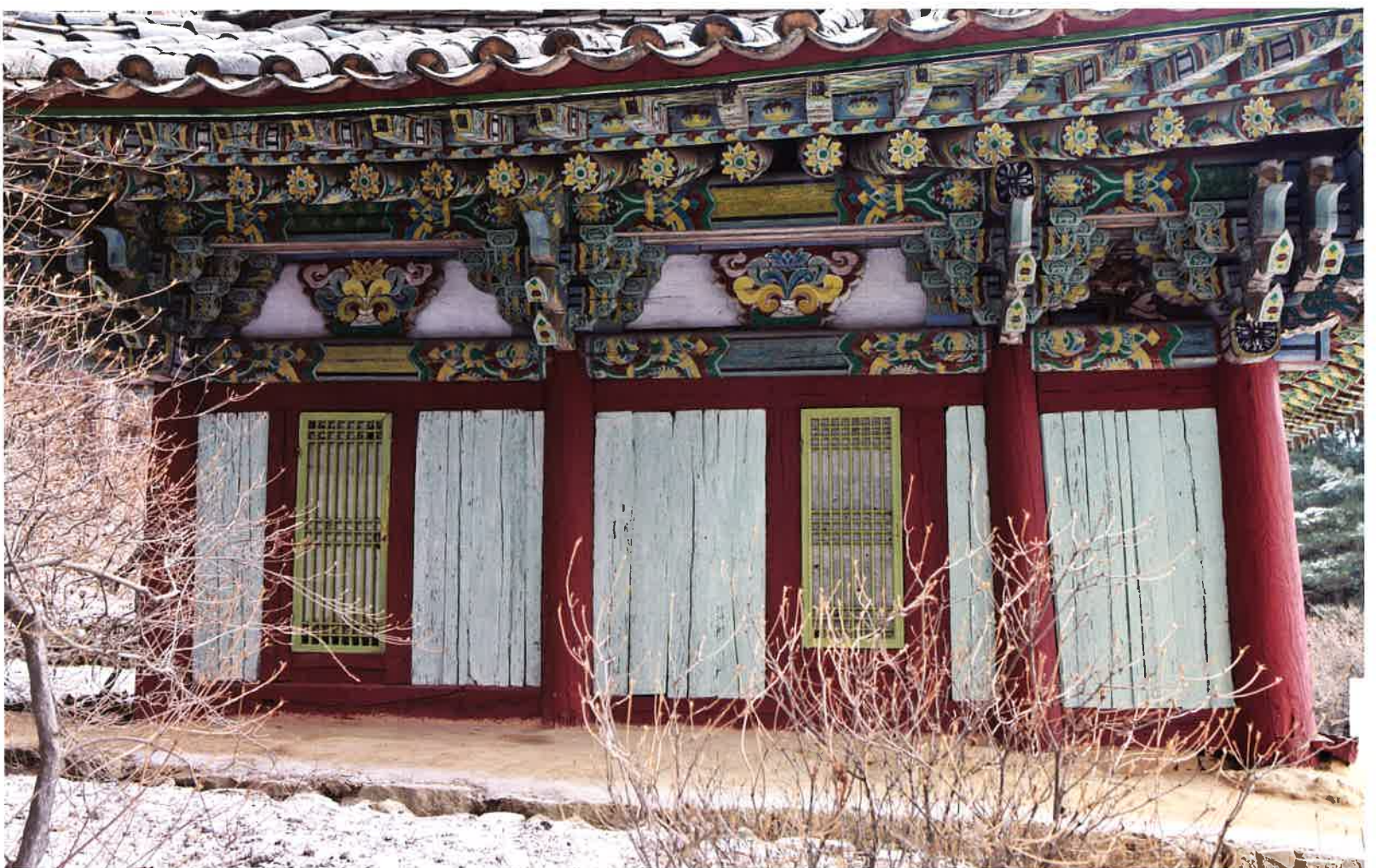
불영암 서쪽 측면 벽체 / 佛影庵 西側 壁體 / western wall, Puryongam
