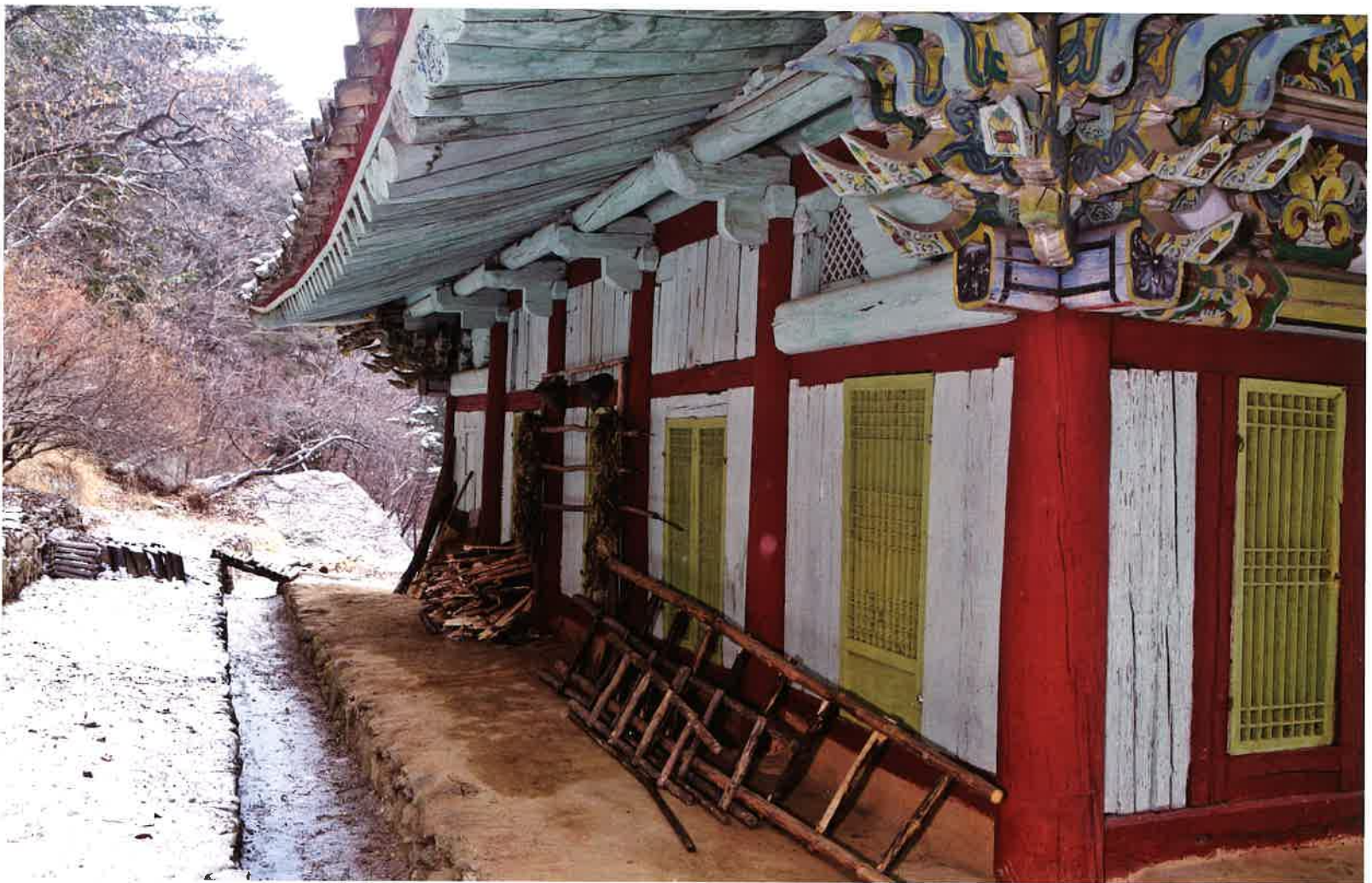
불영암 뒷면 처마와 공포 / 佛影庵 後面 軒·拱包 / backward eaves and brackets, Puryongam
