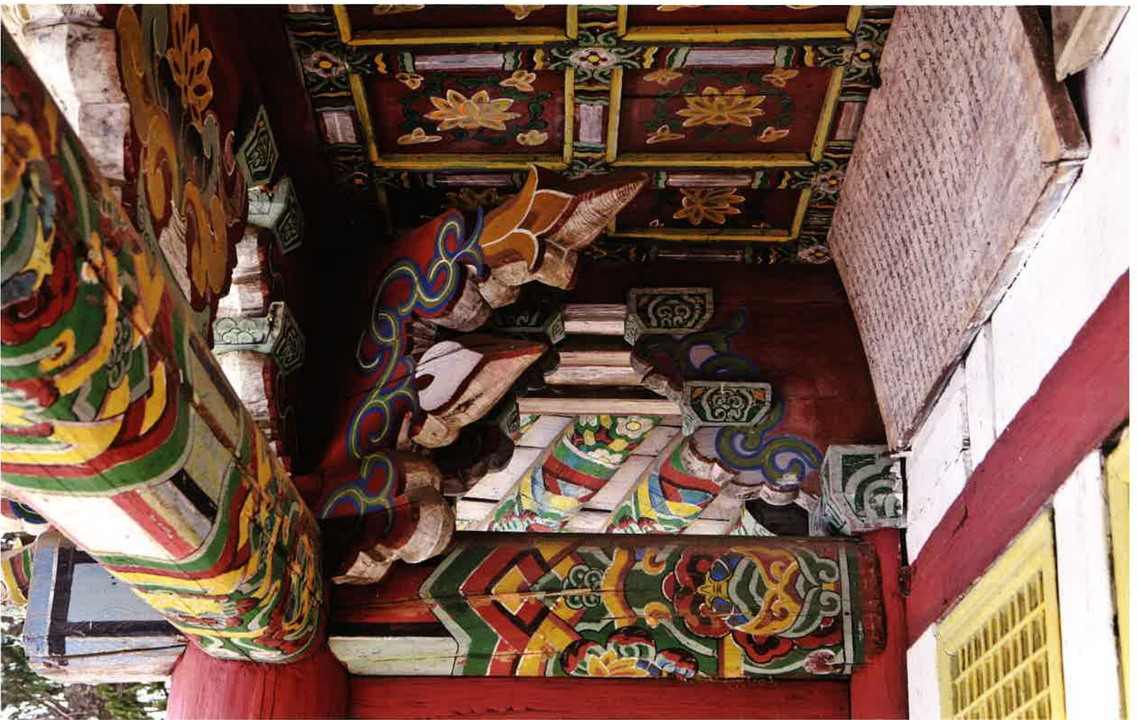
불영암 뒷간 주상포 / 佛影庵 退間 柱上包 / brackets above columns of space with extra poles outside the inner fence, Puryŏngam
