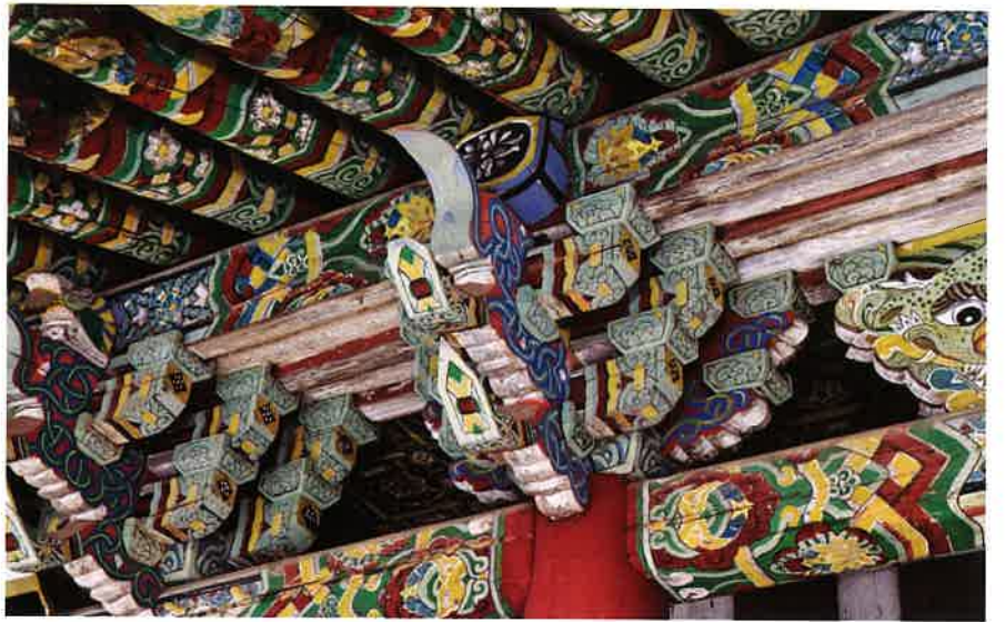
불영암 앞면 주상포 / 佛影庵 前面 柱上包 brackets above front columns, Puryongam
