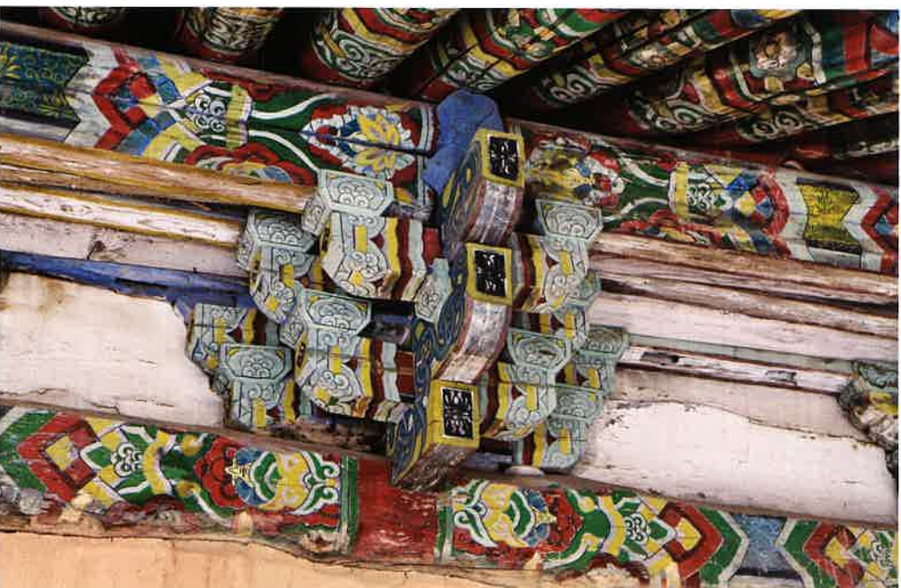
불영암 동쪽 측면 주상포 / 佛影庵 東側 柱上包 / brackets above eastern columns, Puryongam
