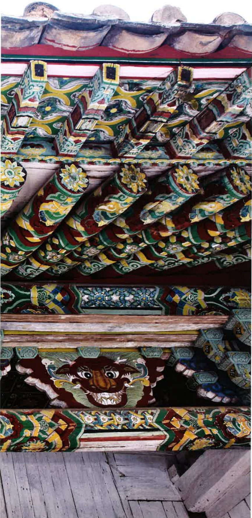
불영암 앞면 액방과 화반 / 佛影庵 前面 額枋·花盤 front lintel and Hwaban, Puryongam
