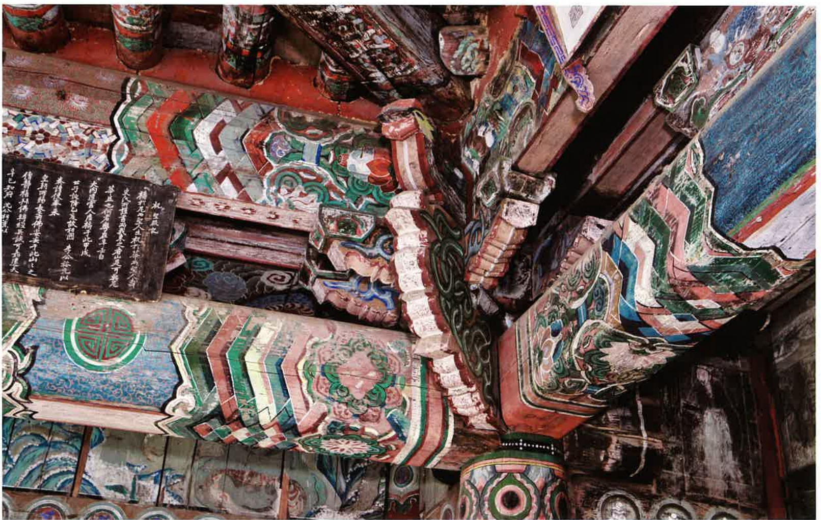
축성전 기본채와 동쪽 날개채 연결 공포 / 祝聖殿 基本架·東側 翼舍 連結 拱包 connecting brackets between main building and eastern wing building, Ch'uksongjŏn hall
