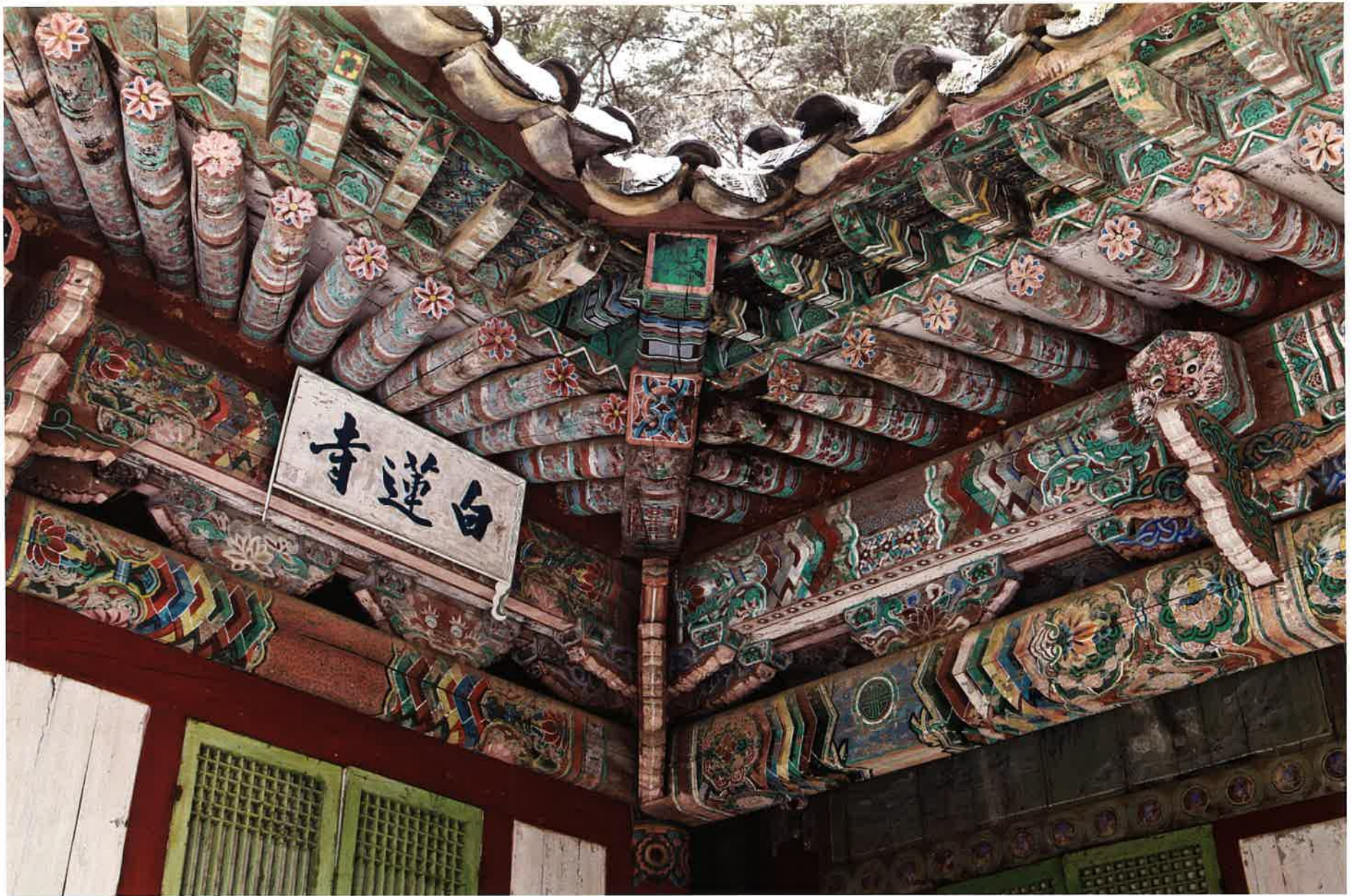
축성전 기본채와 서쪽 날개채 연결구조 / 祝聖殿 基本채·西側 翼舍 結構 connecting structure between main building and western wing building, Ch'uksongjŏn hall
