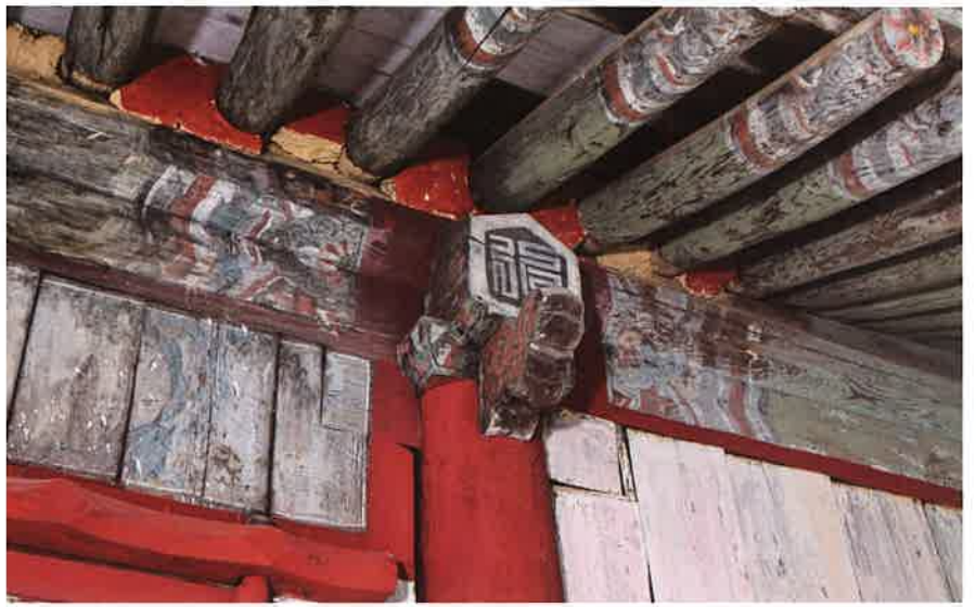
축성전 동쪽 날개채 뒷면 주상포 1 / 祝聖殿 東側 翼舍 後面 柱上包 1 brackets 1 above backward columns of eastern wing building, Ch'uksongjŏn hall
