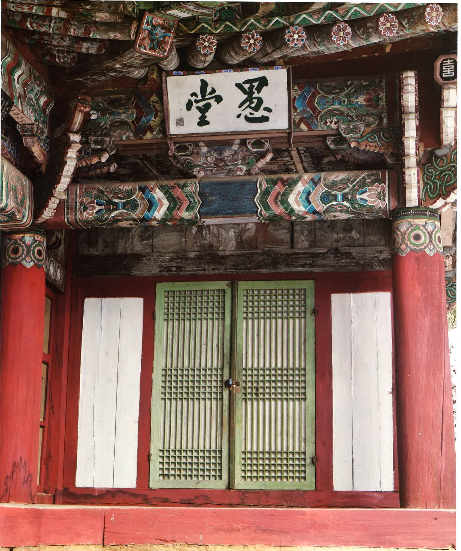
축성전 동쪽 날개재 앞면 / 祝聖殿 東側 翼舍 前面 / front of eastern wing building, Ch'uksongjon hall
