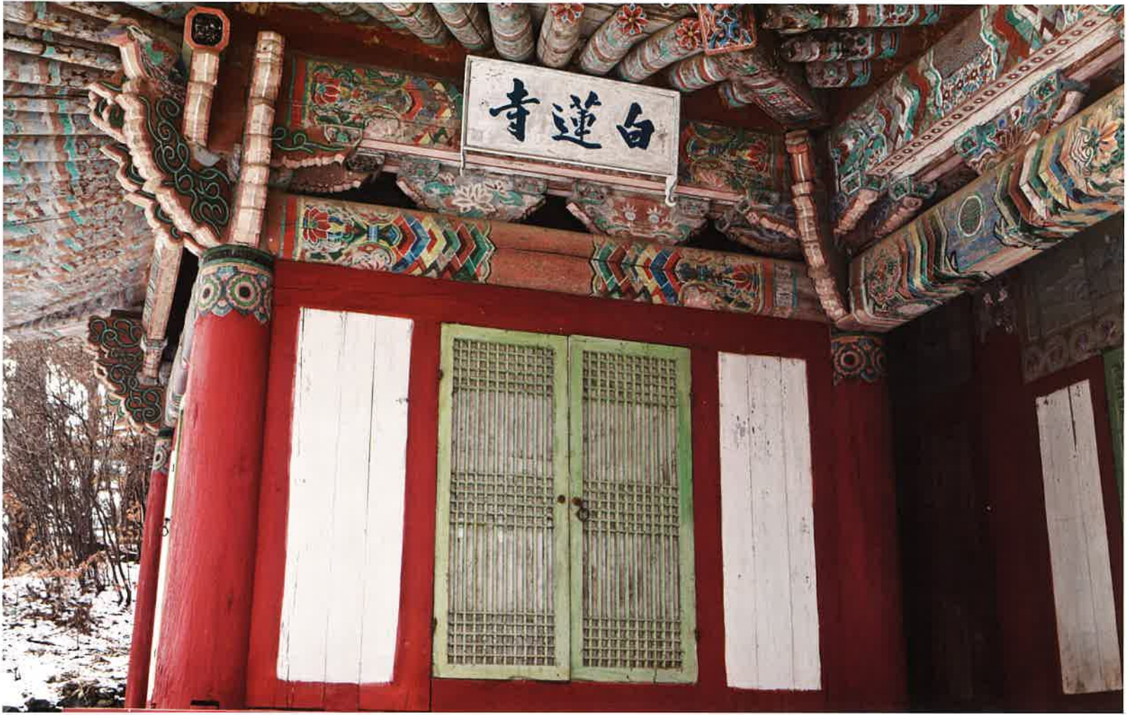
축성전 서쪽 날개채 앞면 / 祝聖殿 西側 翼舍 前面 / front view of western wing building, Ch'uksongjŏn hall
