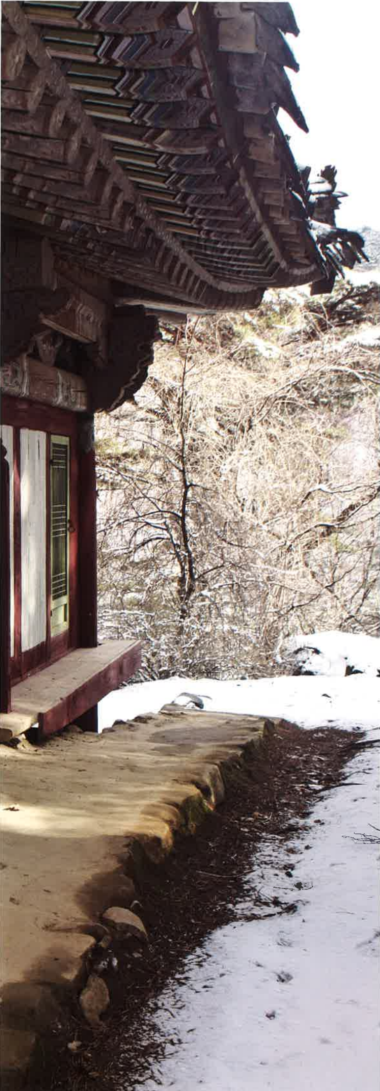
축성전 서쪽 날개채 남쪽 측면 처마와 공포 祝聖殿 西側 翼舍 南側面 軒·拱包 southern eaves and brackets of western wing building, Ch'uksongjŏn hall
