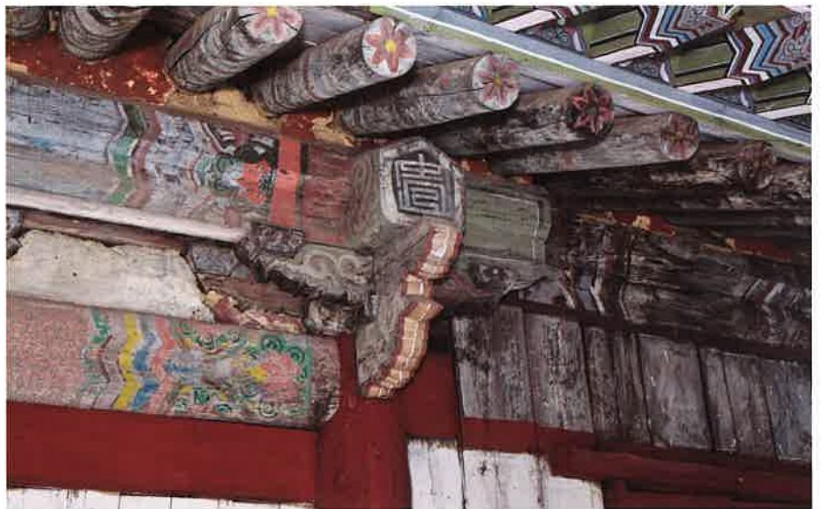
축성전 동쪽 날개채 뒷면 주상포 2 / 祝聖殿 東側 翼舍 後面 柱上包 2 brackets 2 above backward columns of eastern wing building, Ch'uksongjŏn hall
