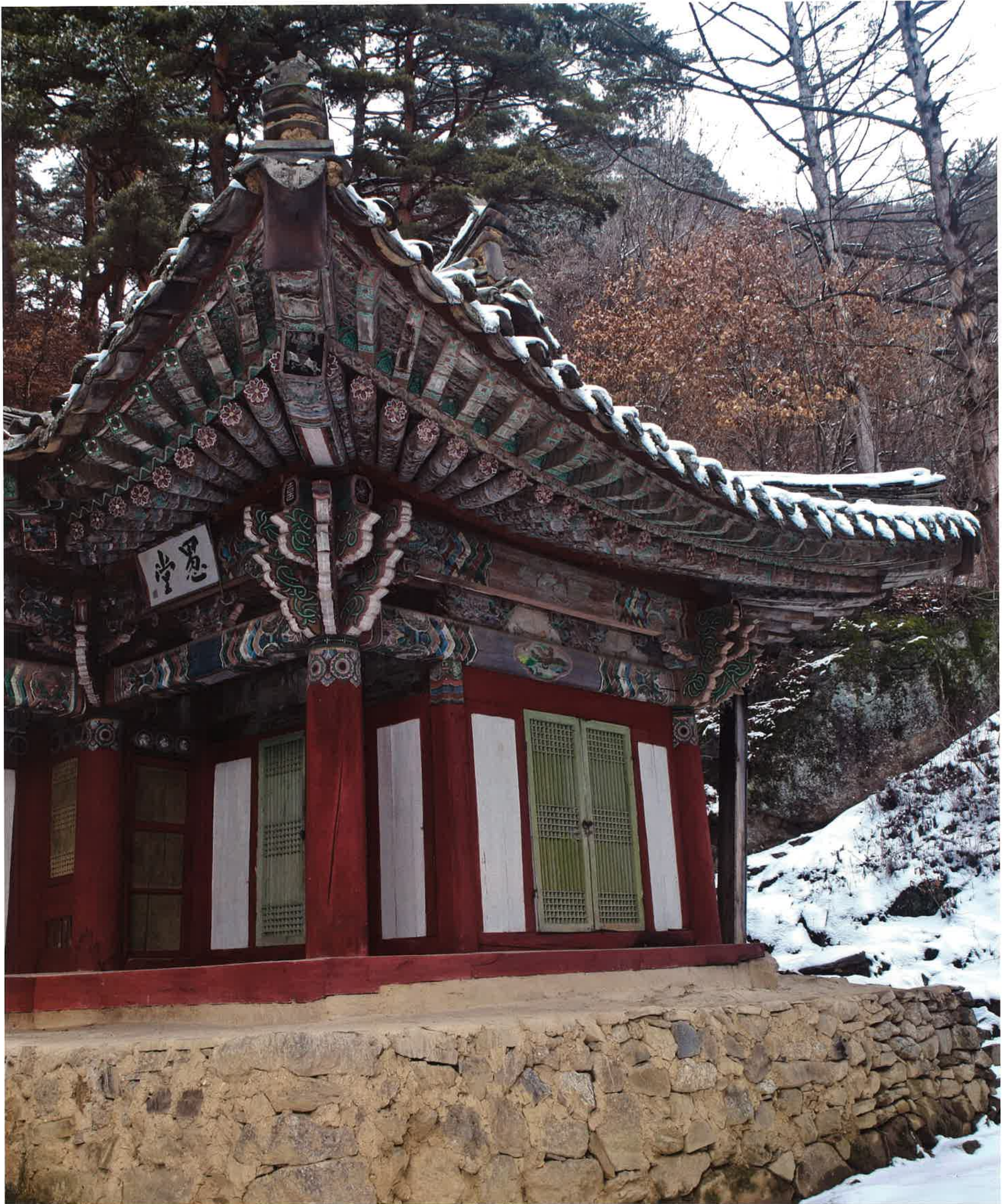
축성전 동쪽 날개채 전경 / 祝聖殿 東側 翼舍 全景 / whole view of eastern wing building, Ch'uksongjŏn hall
