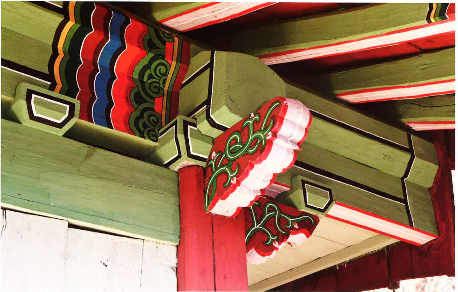
칠성각 귀포 / 七星閣 耳包 / corner brackets, Ch'ilsyongak shrine
