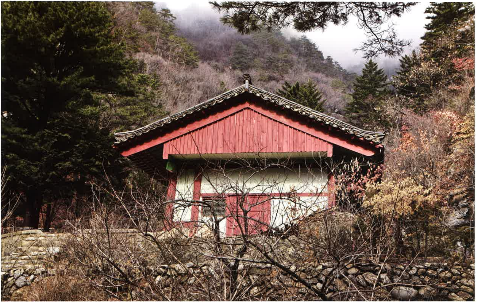
하비로암 본전 동쪽 측면 / 下毘盧庵 本殿 東側面 / eastern side of main hall, Habiroam
