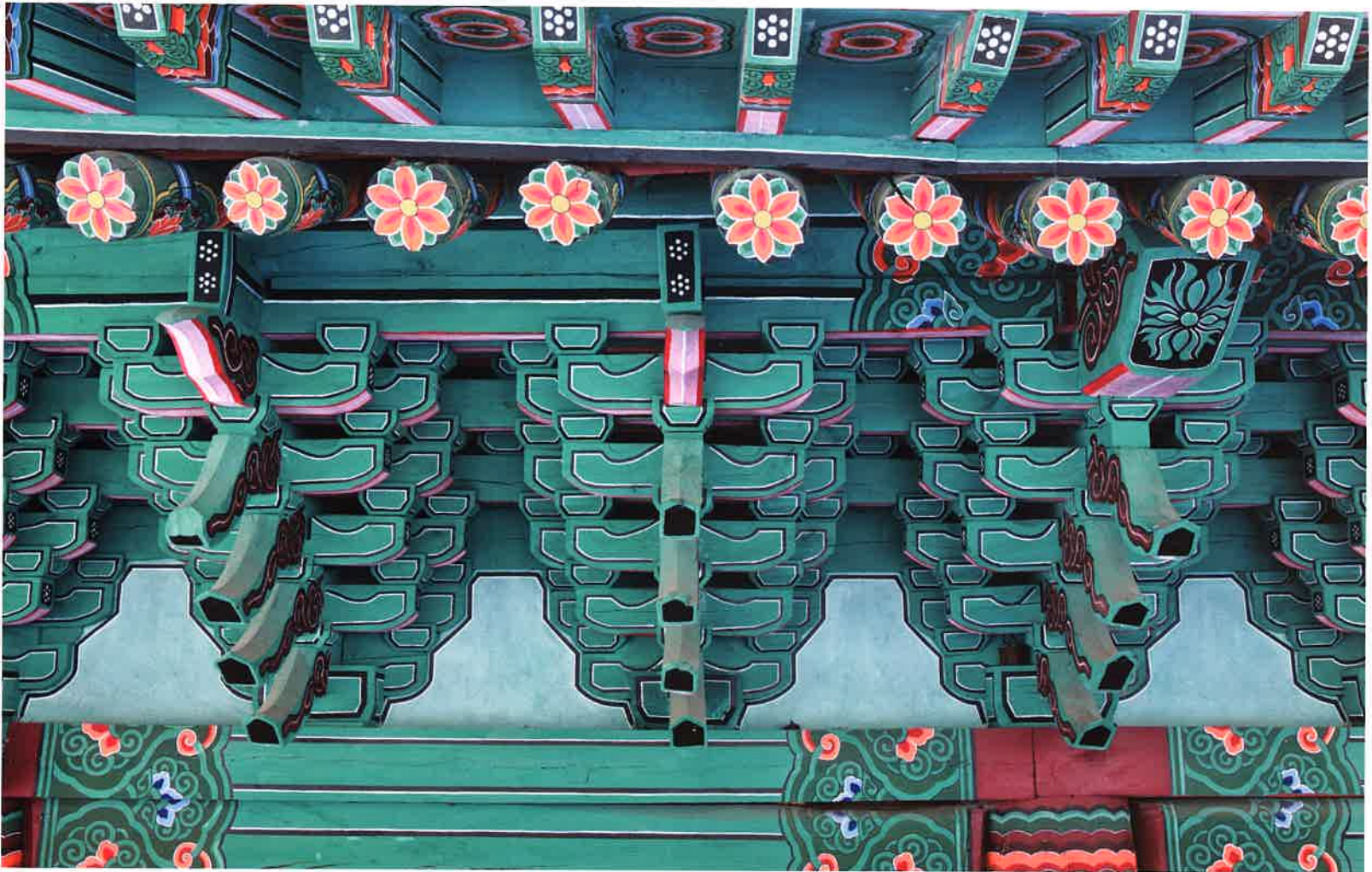
극락전 뒷면 주간포 / 極樂殿 後面 柱間包 / brackets between backward columns, Kūngnakchön hall
