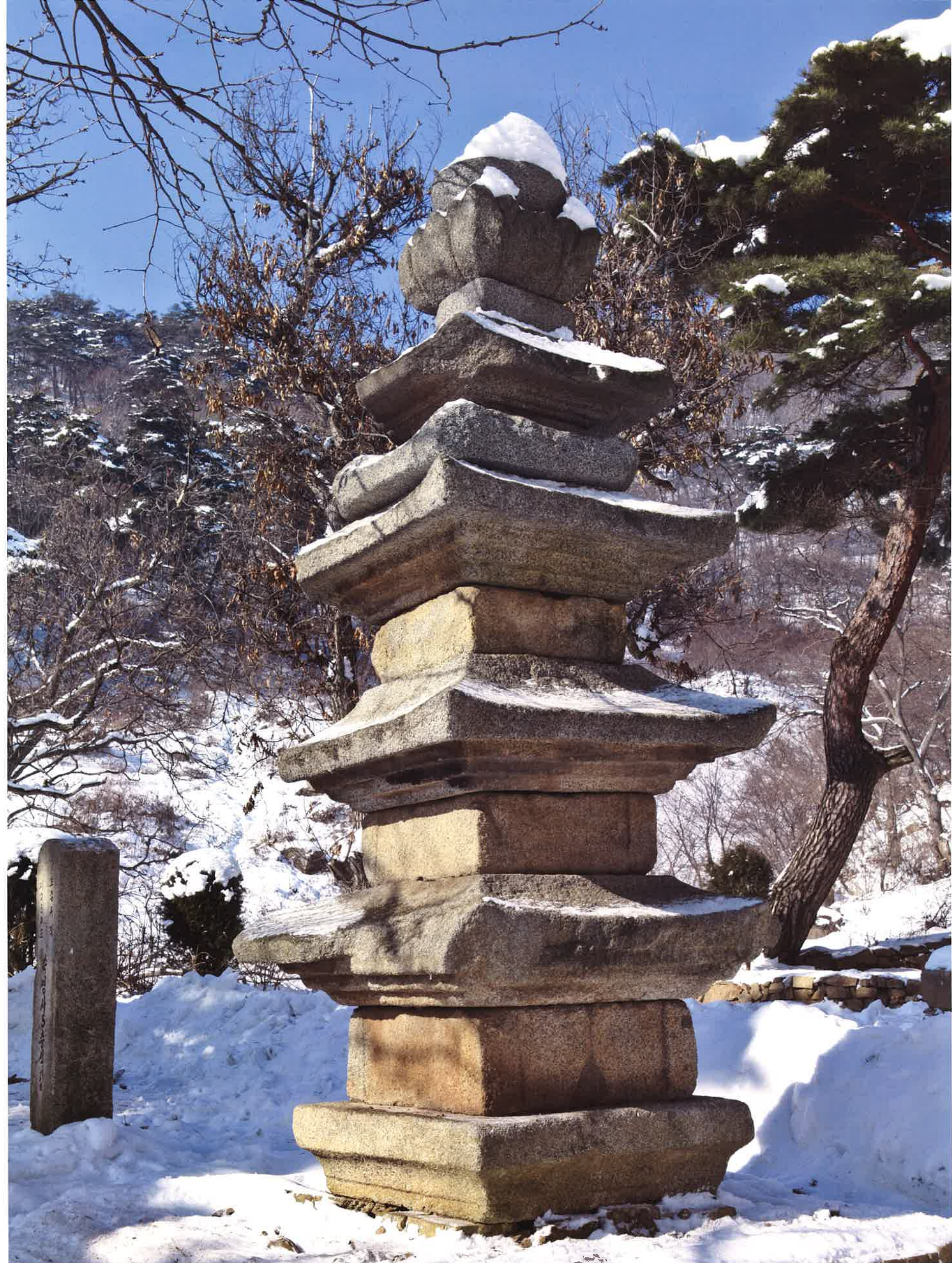
속명사 5층석탑(보존유적 제280호) / 緘命寺 五層石塔 / 5-storied stone pagoda, Songmyŏngsa (as national preserved heritage remains No. 280)
