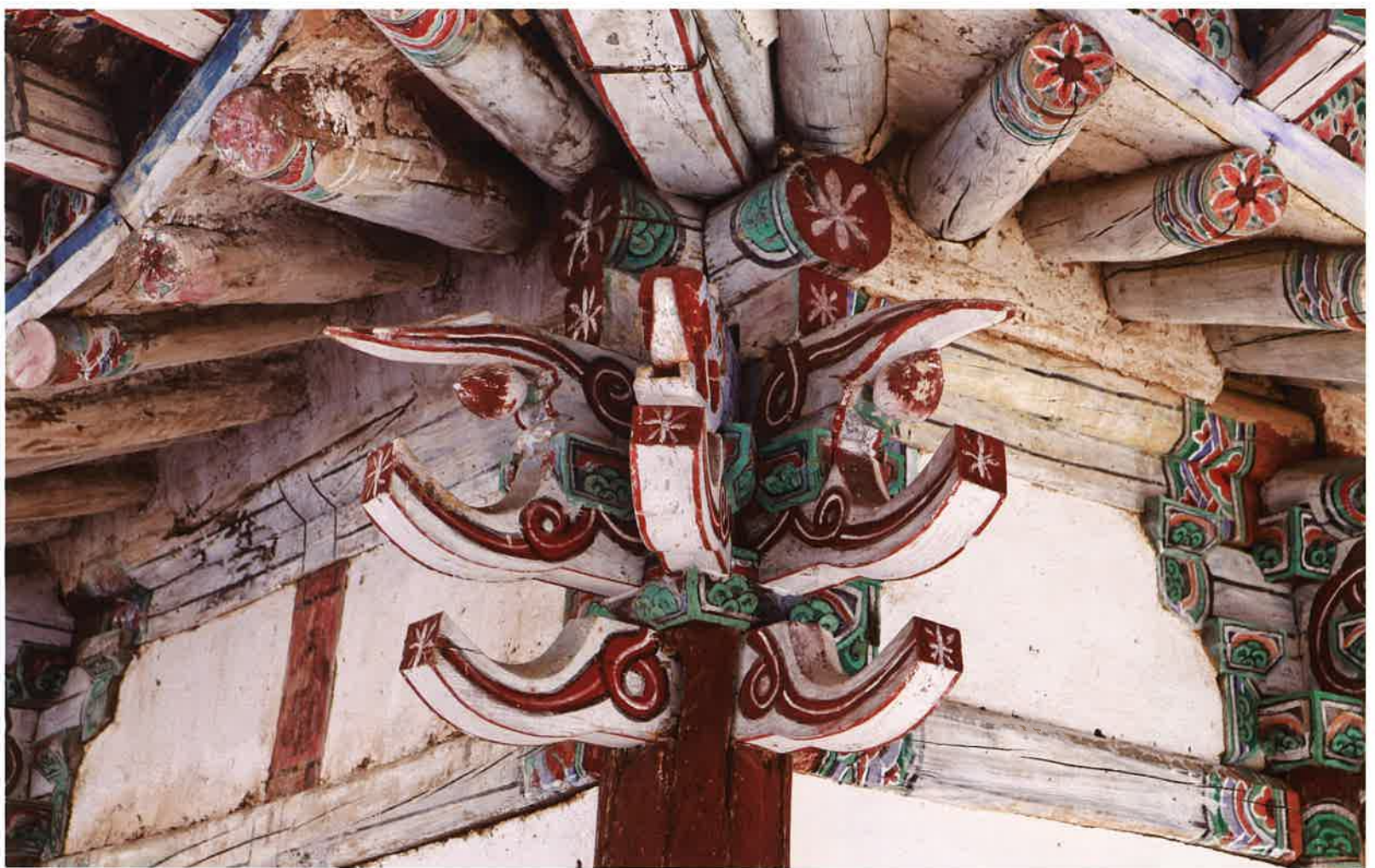
약사전 뒷면 동쪽 귀포 / 藥師殿 後面 東側 耳包 / backward eastern corner brackets, Yaksajön hall
