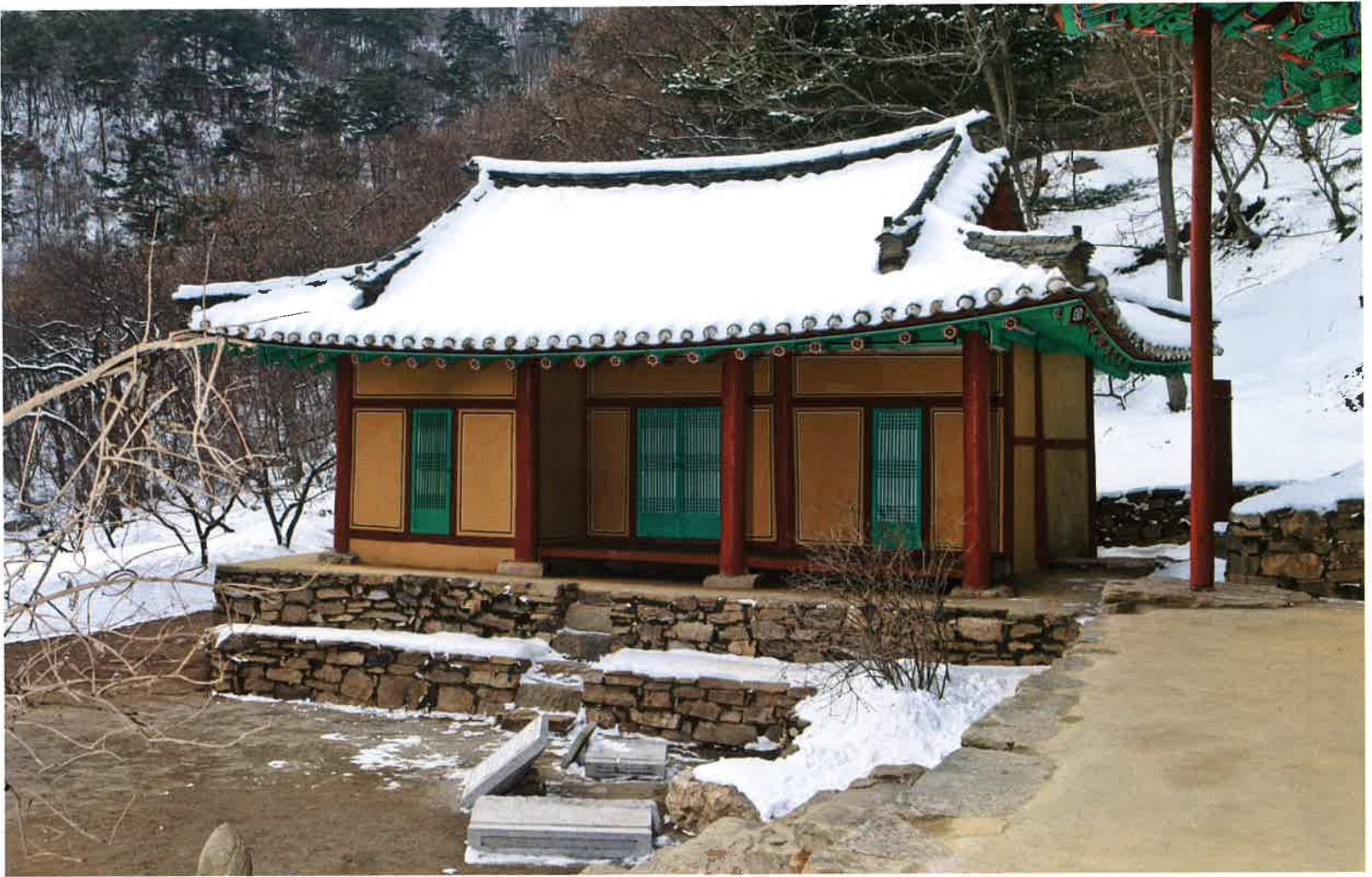
서쪽 요사채 전경 / 西側 寮舍齋 全景 / whole view, western priest's residence
