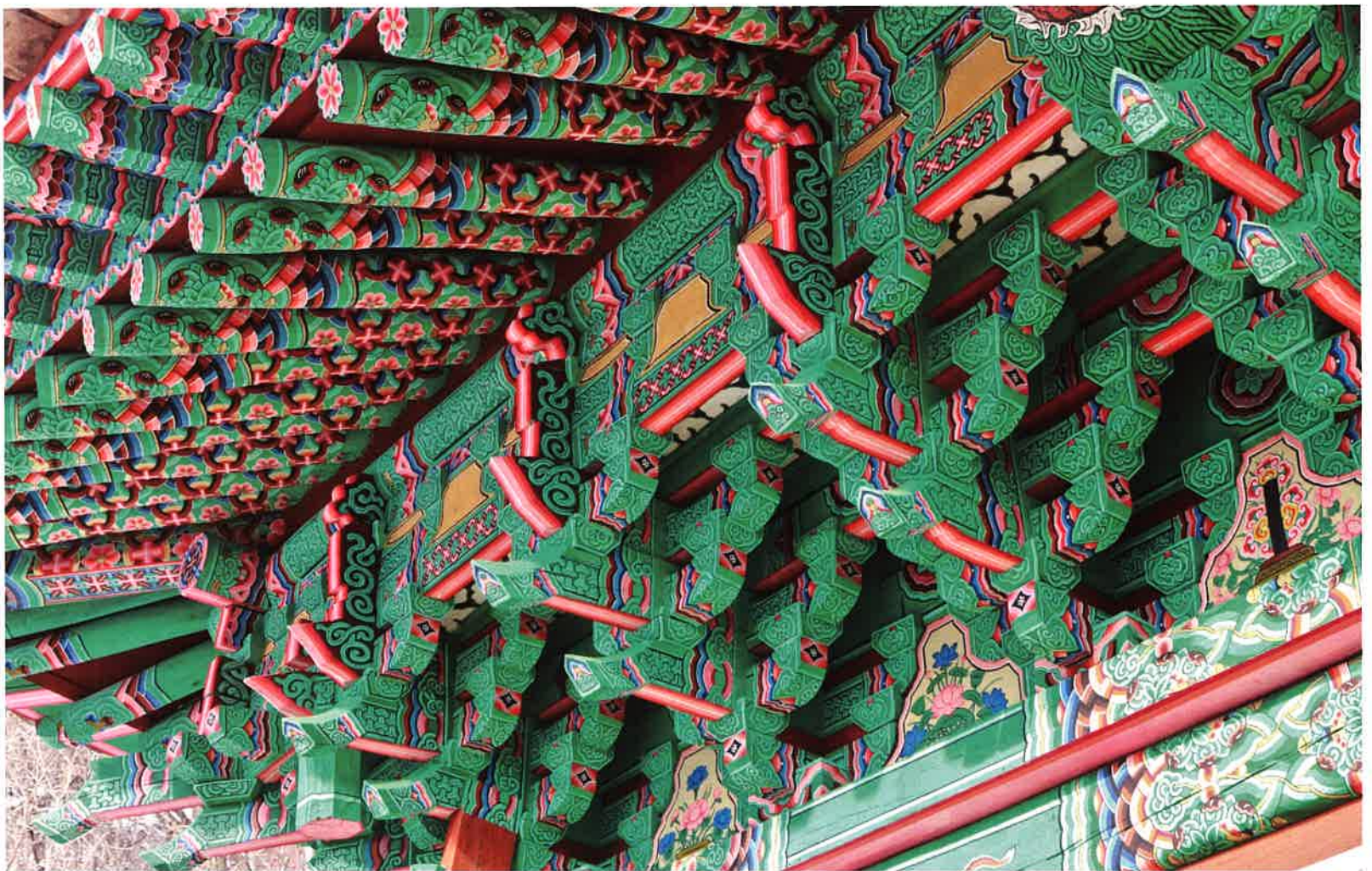
보광전 앞면 귀포 / 普光殿 前面 耳包 / front corner brackets, Pogwangjeon hall
